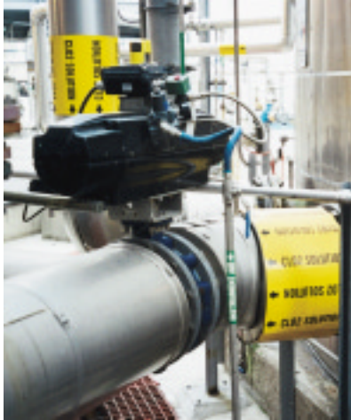
Upper left: DYNACTAIR spring return actuator with lock-out/tag-out, mounted to a 10" ACRIS isolating a CLO2 tank in a pulp mill. Upper middle: Manually operated 8" ACRIS replacing plug valves for pump isolation in EDC and VCM service. Upper right: Manually operated 4" ACRIS for UV light isolation in high purity water.
